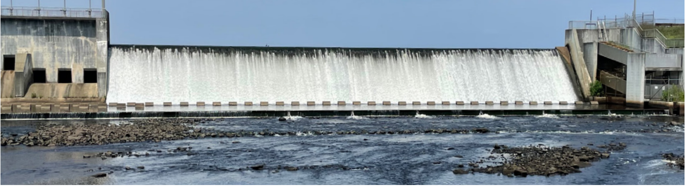
Union Lake Dam
