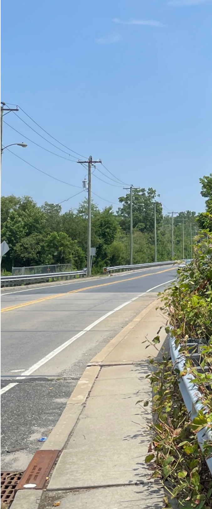
Sharp Street has a high crash density and serves as the access point to Riverview Park in Millville.
