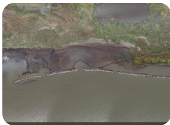
① Basket Flats hybrid breakwaters Source: American Littoral Society
