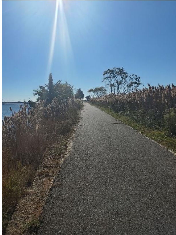
Figure 8: Earth Dike Bike Path in Maurice River Township (photo source: Alltrails)
