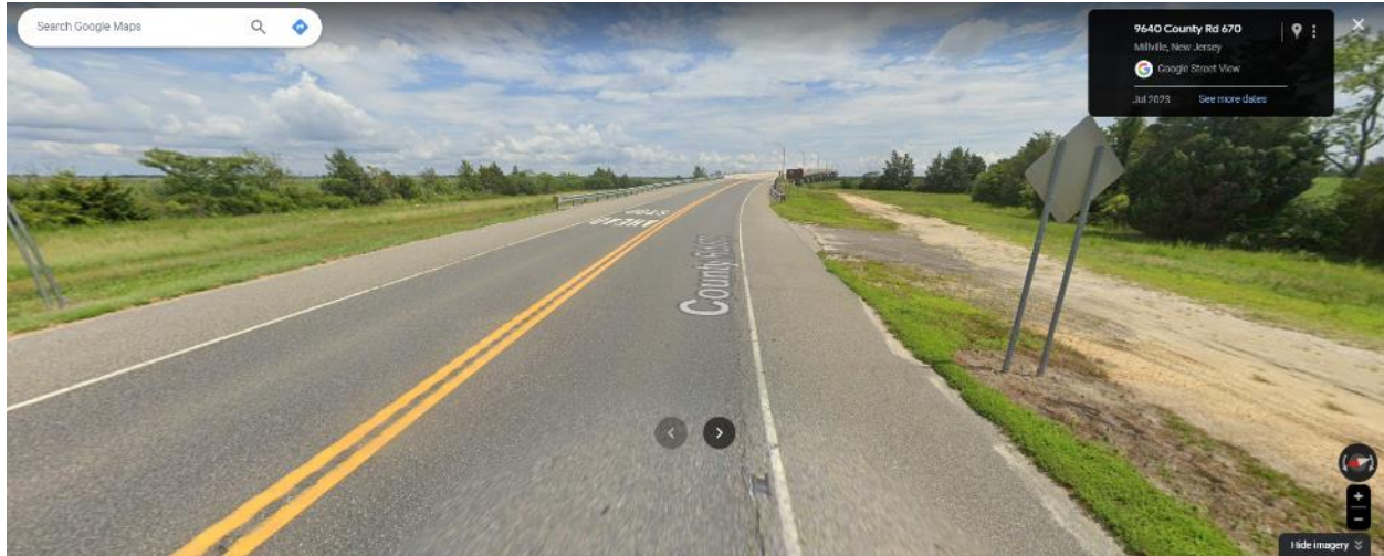
Figure 7: CR 67 Approaching Mauricetown Bridge
