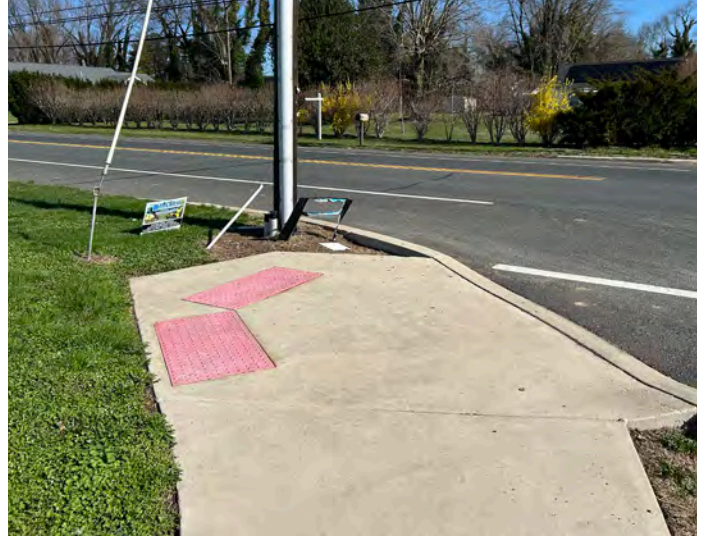
AD-2: ADA ramp at Cassidy Court and Shiloh Pike
