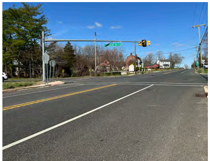
AD-6: Intersection of Shiloh Pike and Barretts Run Rd
