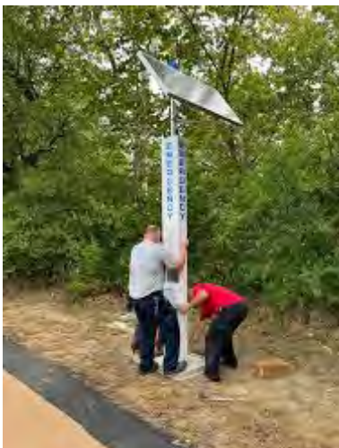
Figure 71: Blue light call station
