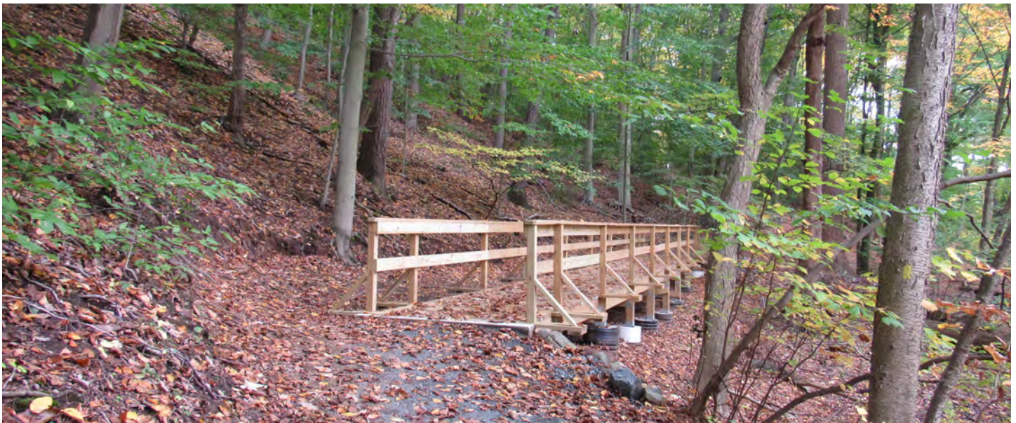
Figure 74: Boardwalks can be used in ecologically sensitive areas to minimize disturbance and impacts to hydrology, Image Credit: AKRF
