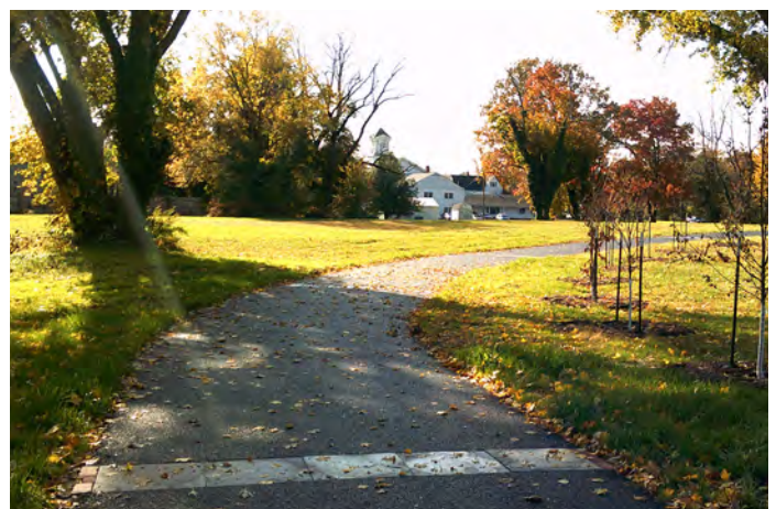
Figure 61: Porous Asphalt Trail in Allentown, New Jersey, Image Credit: AKRF
