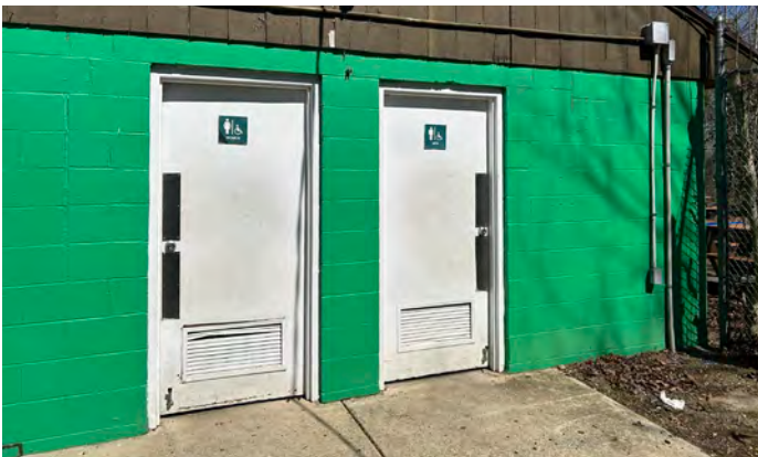
Figure 46: Existing restroom at Cohanzick Zoo, Image Credit: AKRF
