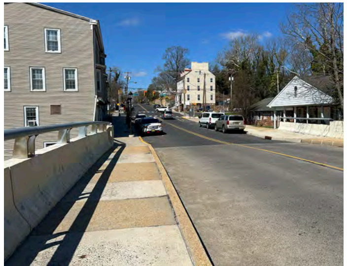
AD-30: Commerce St. Bridge
