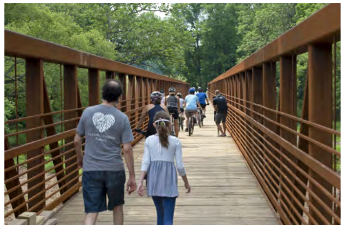
Figure 59: Stony Brook Pedestrian Bridge at Mercer Meadows in Mercer County, New Jersey, Image Credit: AKRF
