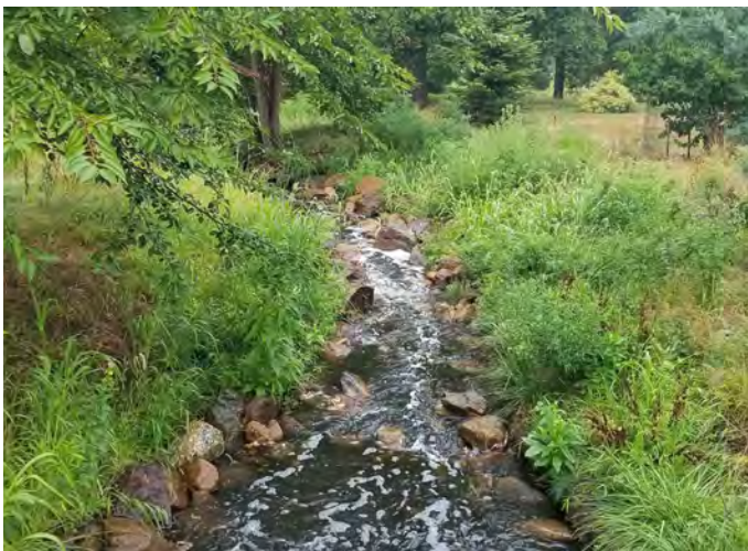
Figure 65: Streambank stabilization, Image Credit: AKRF
